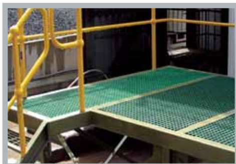
Concrete batching plant, Busselton, WA
