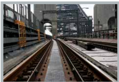
Sydney Harbour Bridge rail walkway
