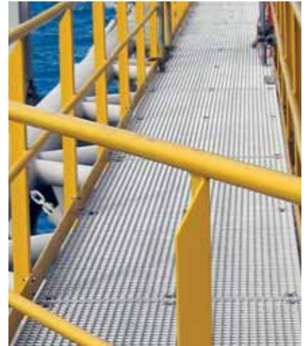
Weldlok® aluminium grating at Abbot Point Coal Terminal, QLD
